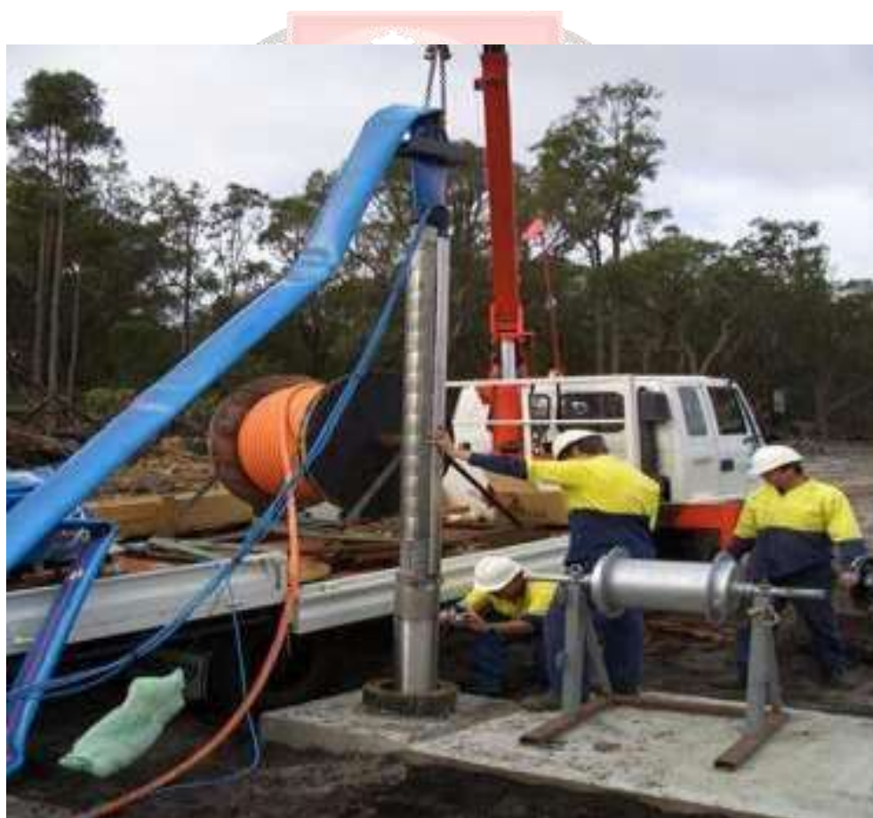
Fig. 5: Hydraulic operated submersible motor lifting machine.
